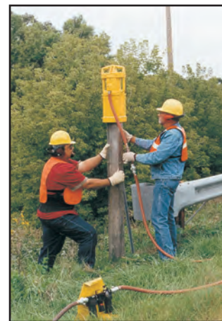
6" x 6" Master Chuck (P/N 070761) Attached for square wood pile.
