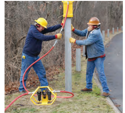
Additional Filter-Regulator - Lubricator recommended with the PD-200G increases tool-life.
