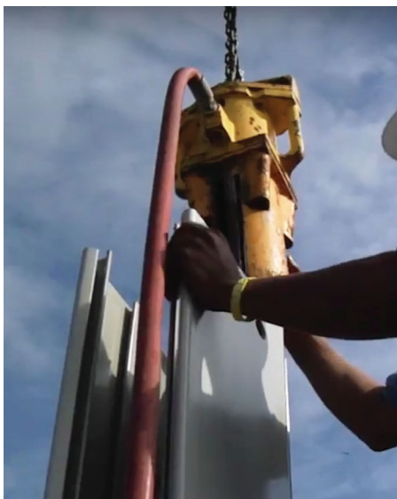
PD-140S driving Truline Vinyl Sheet Pile®
